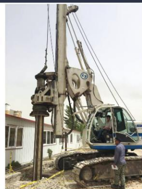
配套土力钻机现场施工 Supporting to SOILMEC Rotary Drilling Rig
