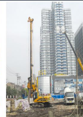
配套福田钻机现场施工 Supporting LOVOL rotary drilling rig
