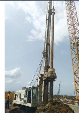
配套迈特钻机现场施工 Supporting to MAIT Rotary Drilling Rig
