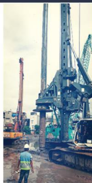
配套利勃海尔钻机现场施工 Supporting to LIEBHERR Rotary Drilling Rig
