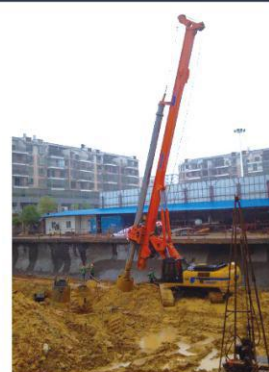
配套九五钻机现场施工 Supporting JOVE rotary drilling rig
