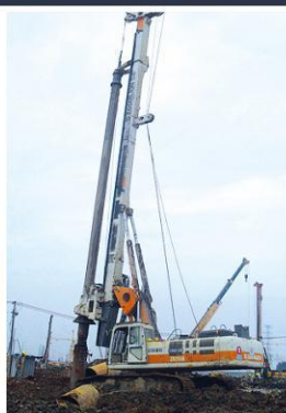
配套中联钻机现场施工 Supporting ZOOMLION rotary drilling rig
