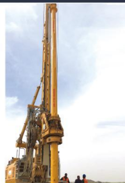
配套宝峨钻机现场施工 Supporting to BAUER Rotary Drilling Rig
