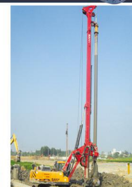
配套三一钻机现场施工 Supporting SANY rotary drilling rig
