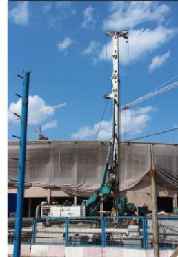
配套卡萨诺蓝地钻机现场施工 Supporting CASAGRANDE rotary drilling rig
