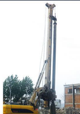
配套中车钻机现场施工 Supporting CRRC rotary drilling rig
